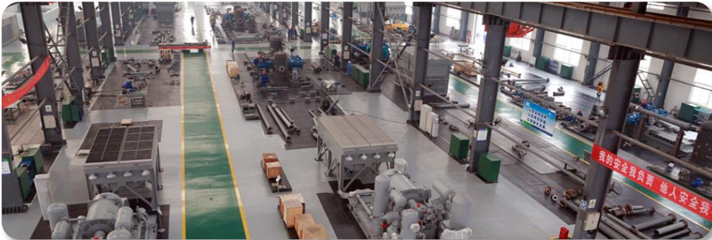
Natural Gas Compressor Industrial Park
