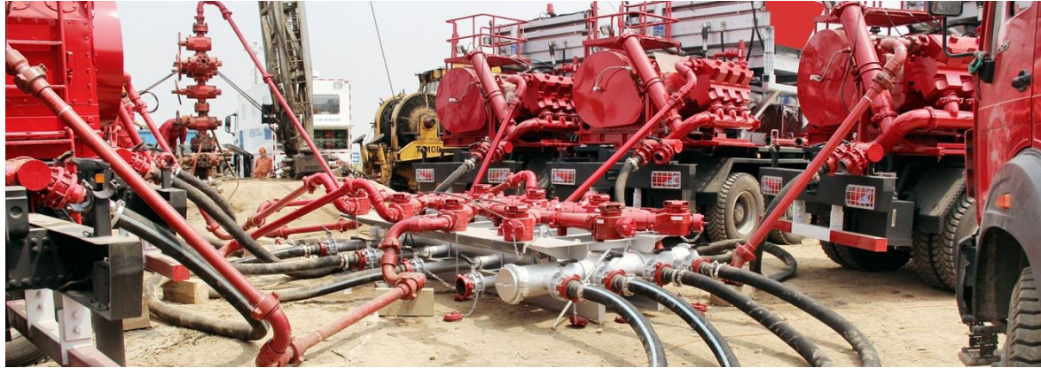
Fracturing Crew Working Site
